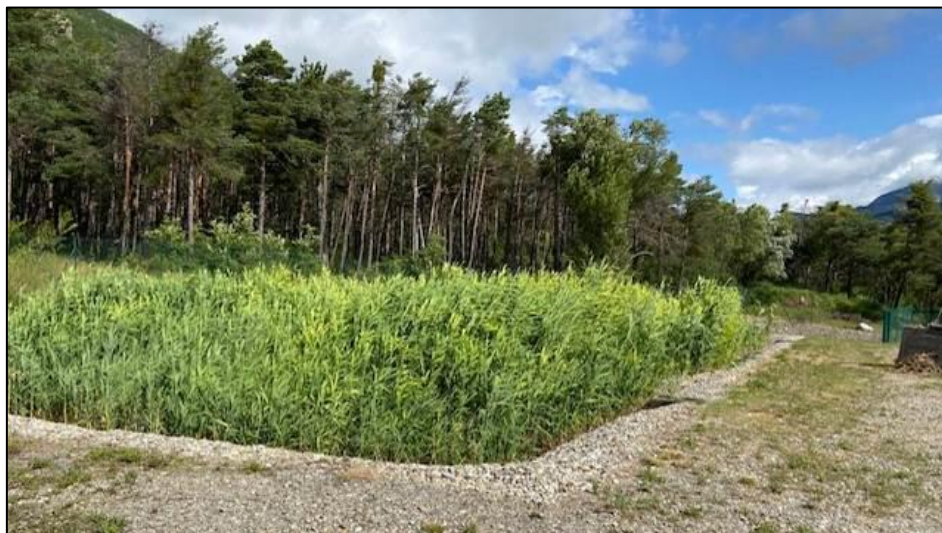
Figure 11: Station d'épuration de Cros
