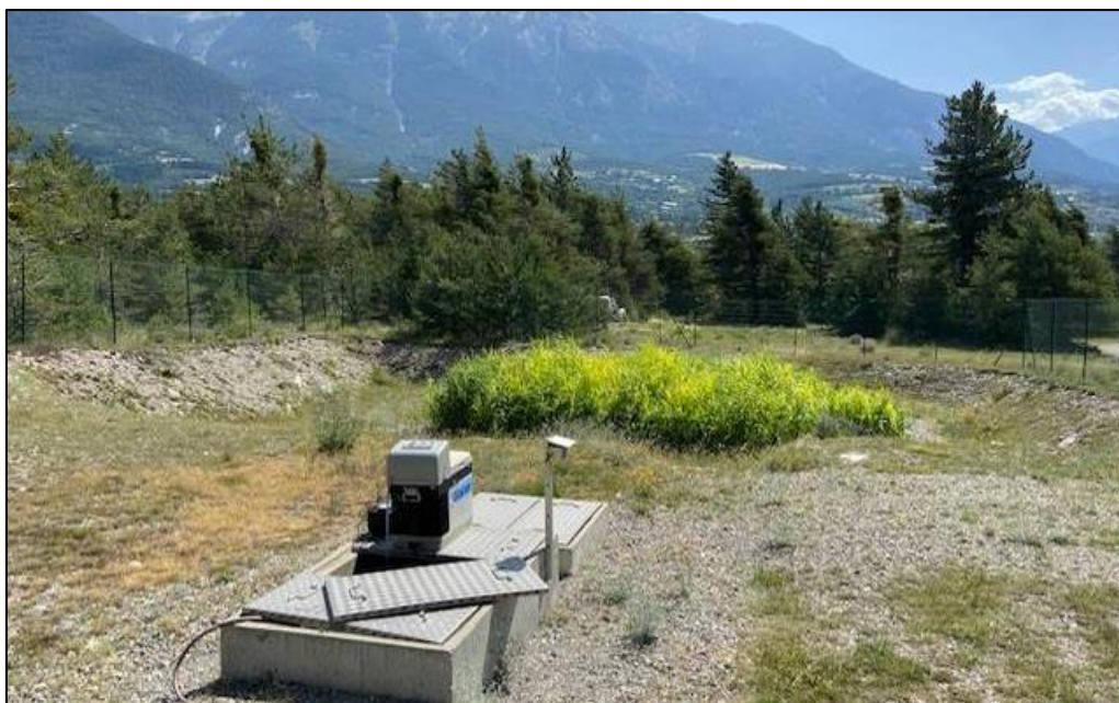
Figure 14: Station d'épuration de St Thomas
