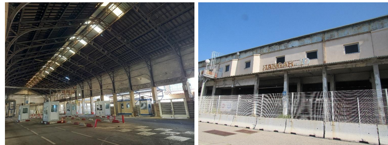
Figure 20 : Hangars, A. Barateau © EODD 2024
