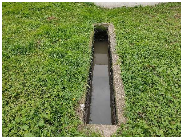
Figure 36: canal de comptage
