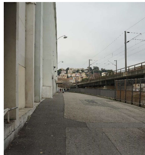
Figure 14 : Photo façade Nord
