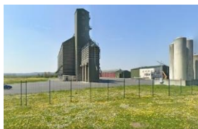
Figure 14: Silo Agora Amblainville - source Agora
