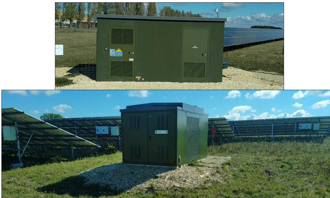
Figure 28 : Illustrations photographiques des structures (source : COMIREM SCOP)
