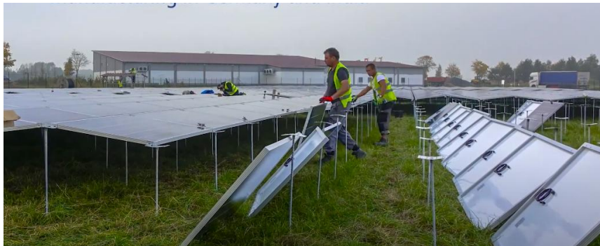
Figure 2 : Installation de la structure (2/2)
