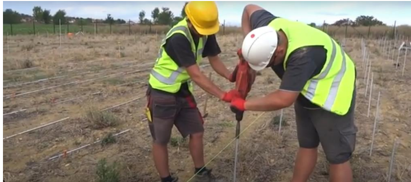
Figure 1 : Installation de la structure (1/2)
