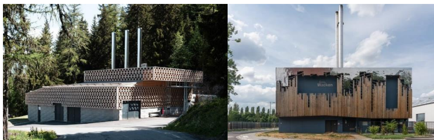
Figure 44 : Exemples de chaufferies biomasse collectives
