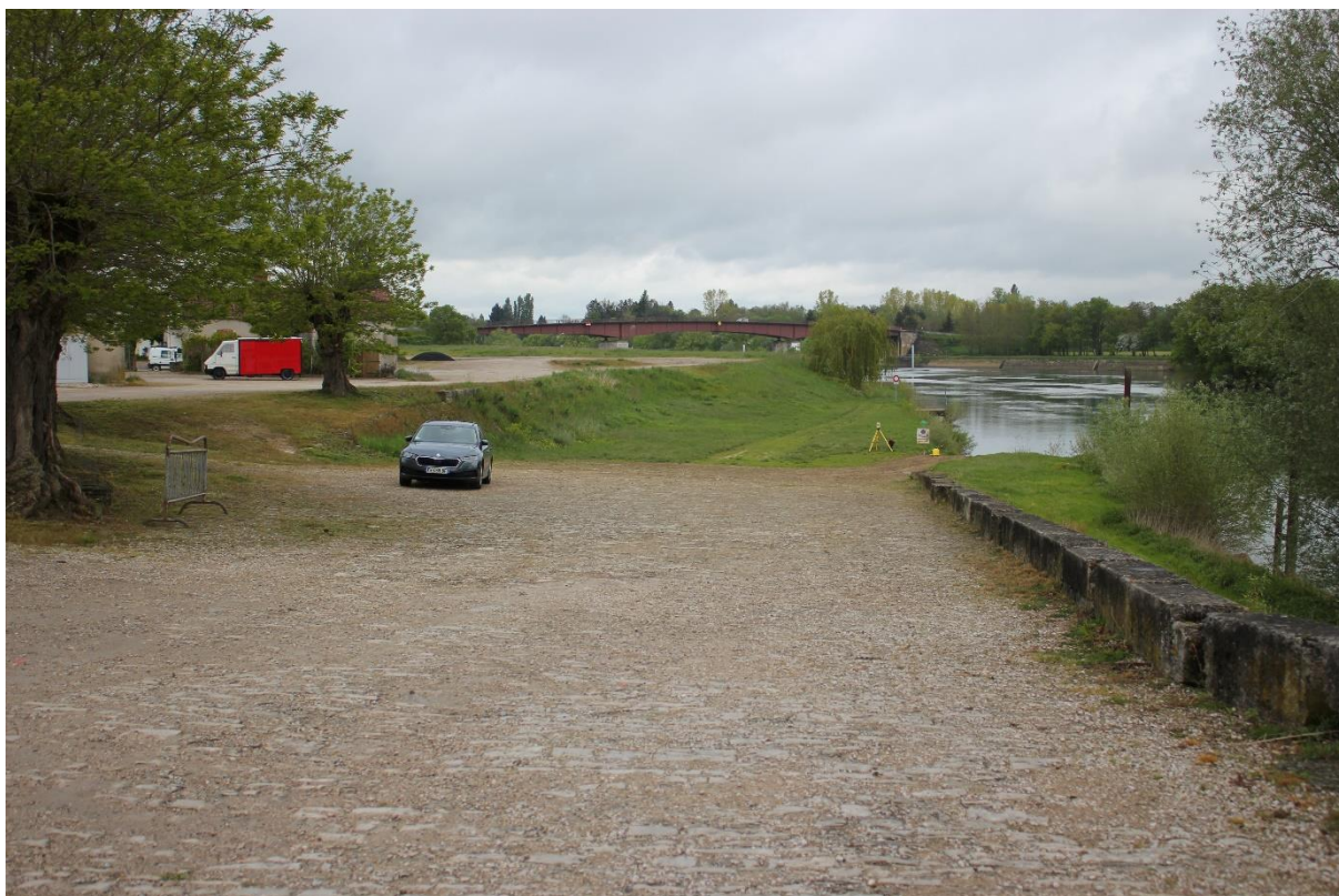
vue parking (direction aval)
