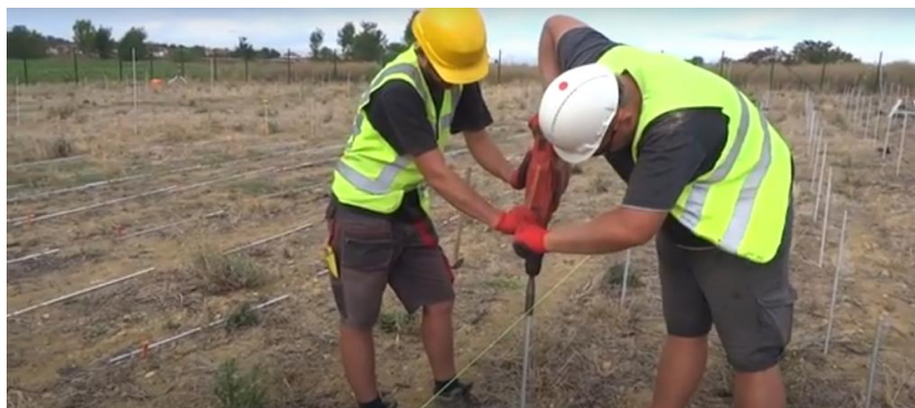
Figure 1 : Installation de la structure (1/2)
