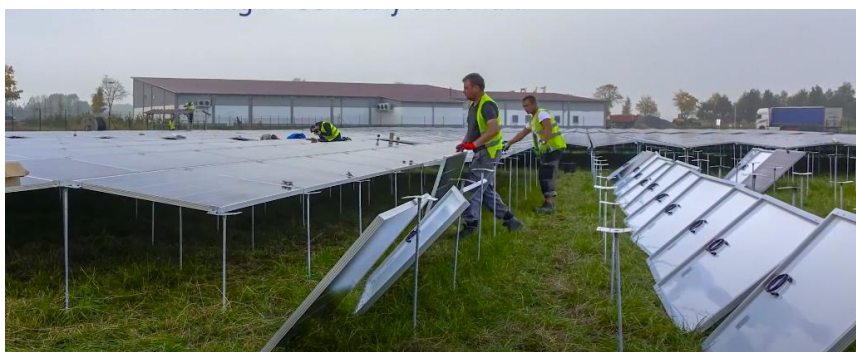
Figure 2 : Installation de la structure (2/2)
