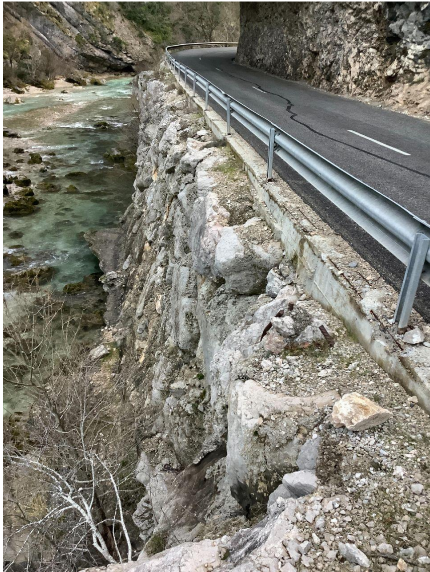
Photo 3 – Mur 1-vue de dessus – BOAS – 09/2021
