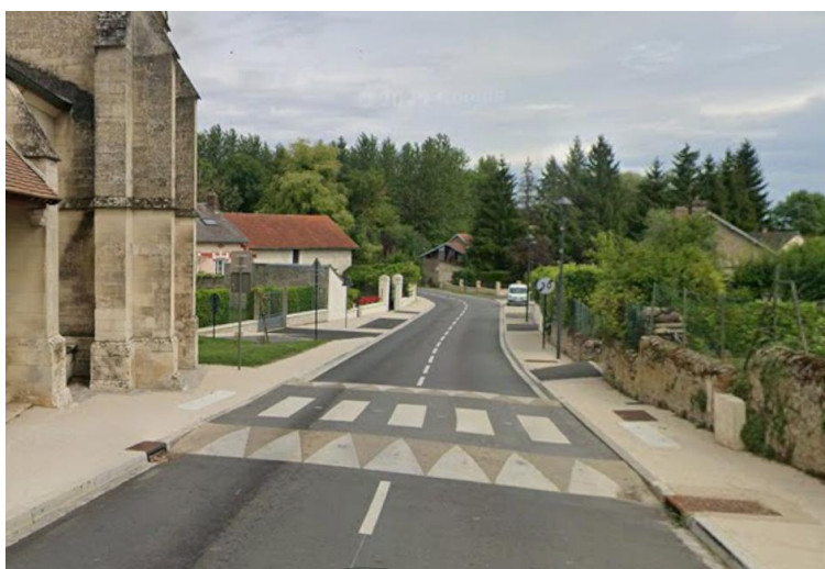
Figure 19: Avaloirs rue de Laon (Altereo - 2025)
