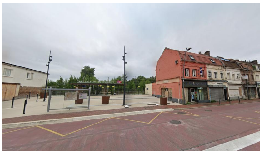
Figure 6: Illustration de l'état existant
