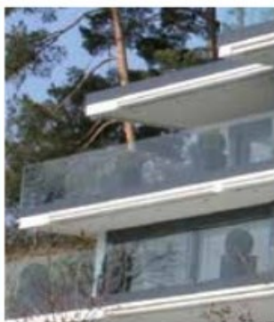
Balustrade de balcon
