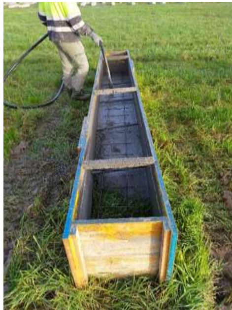
Figure 17 - Coulage des fondations.
