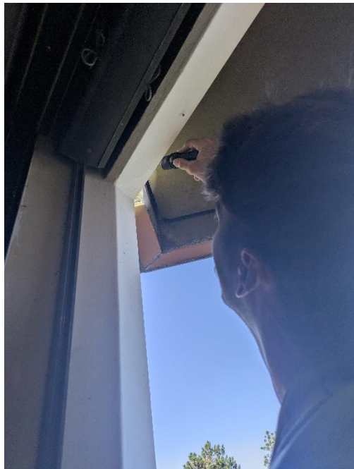
Figure 37 : Inspection des balconnets
