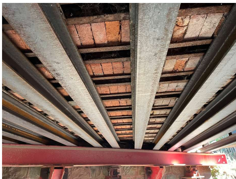
Figure 5 : Photo CFPON 015 – Intrados conforté provisoirement
