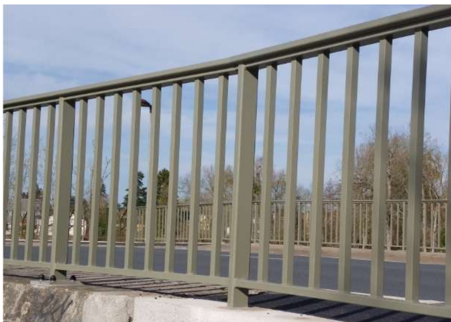
Figure 25 : Garde-corps type S8
