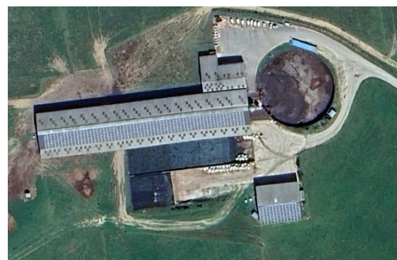
Figure 3 installation photovoltaïque du GAEC
