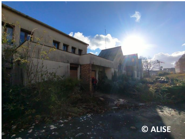
Photo 4 : Façade Est. Laboratoires (photo sur site)
