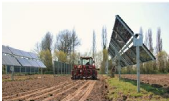
Trackers photovoltaïques (configuration retenue)
