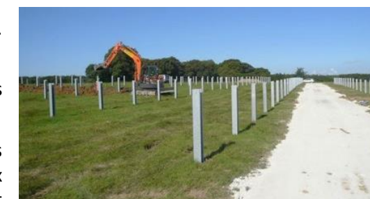
Pose des structures porteuses
