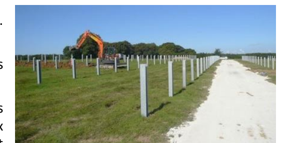
Pose des structures porteuses
