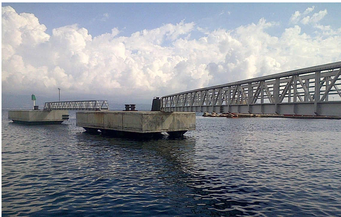
Figure 39 : Passerelle de lamanage [source CCI 2A]
