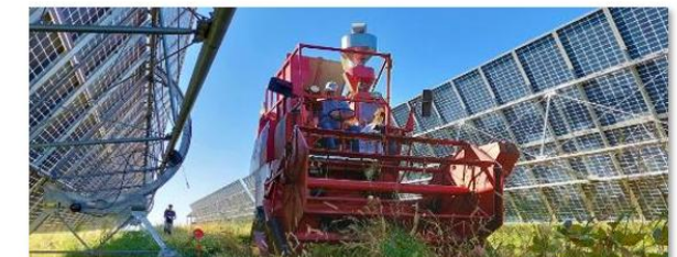
Moncrebeau (47) – 11 MWc – Centrale agrivoltaïque
