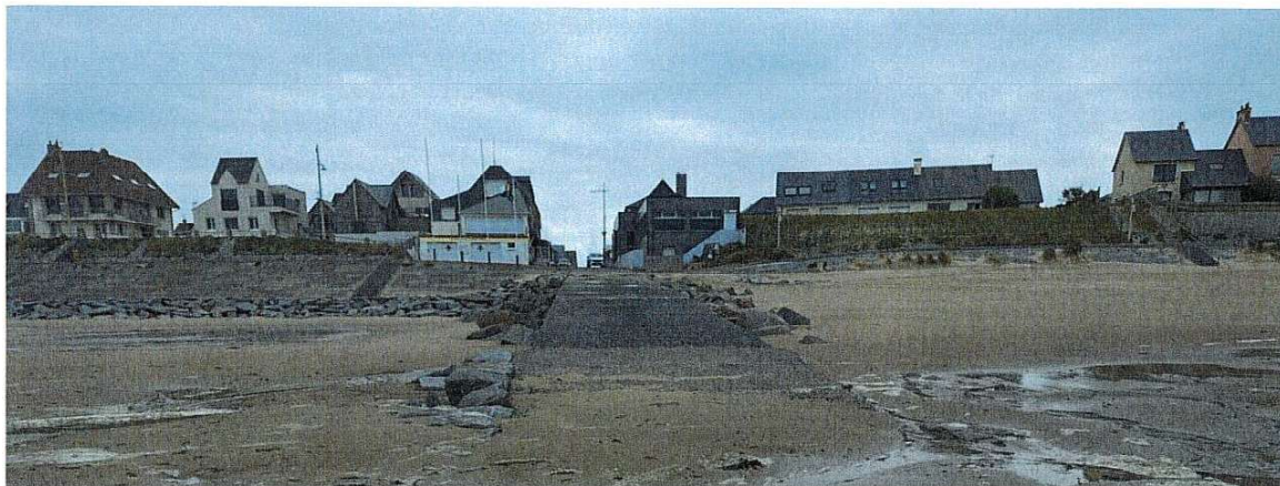
Figure 41 : Photo cale nord. Source : ARTELIA
