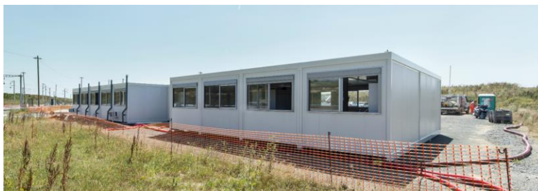
Figure 17 : Installation de la base vie (Source : Cougnaud Services)
