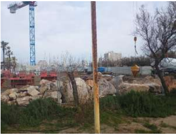
FIGURE 28 : ZONE DE CONSTRUCTION
