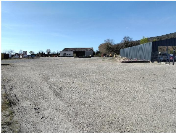
ESPACES BETONNES DEDIEES A LA CIRCULATION
