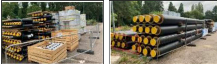
Figure 49 : Stockage des tubes
