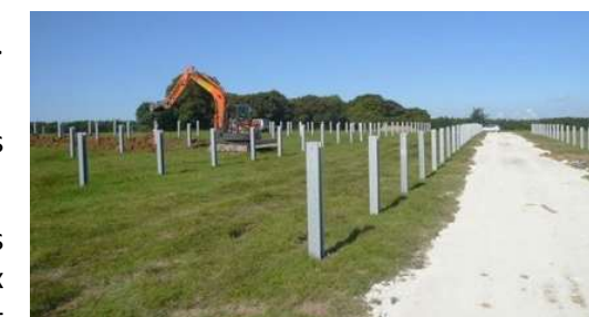
Pose des structures porteuses
