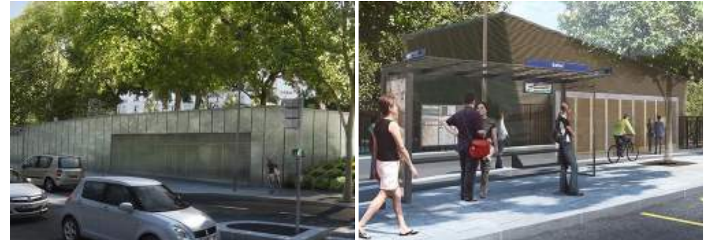
Figure 4. Exemples de locaux techniques (Tram 3)
