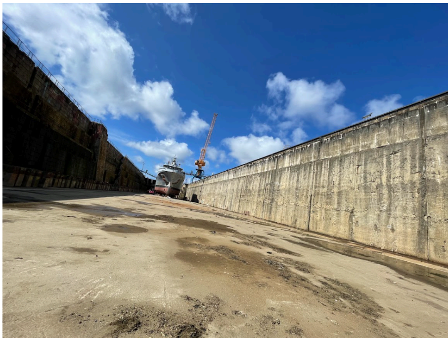
Figure 2. The assembly site. Dock "Form 1" at Brest Port.
