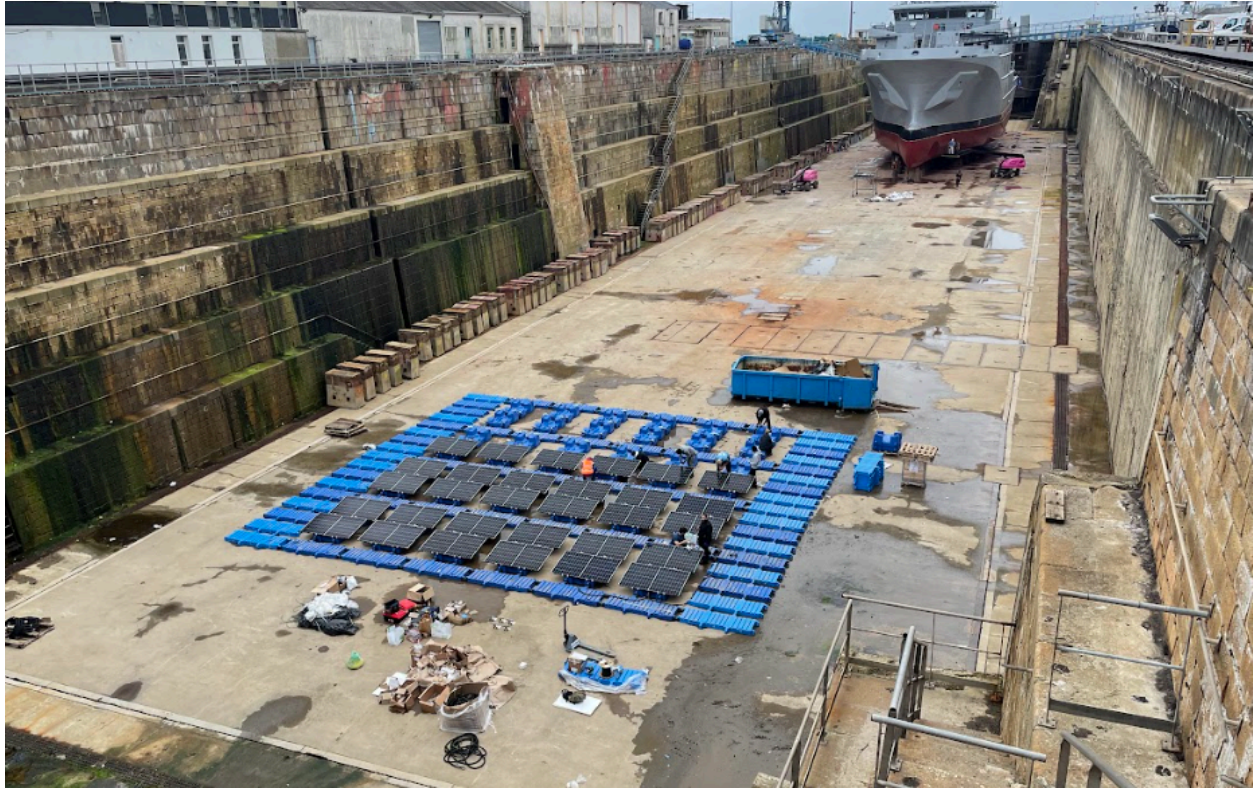
Figure 1. Mounting PV panel on the floaters
