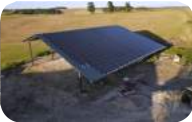
Construction hangar PV – Puylaurens (88)
