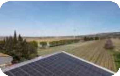
Construction hangar PV – Cruscades (11)
