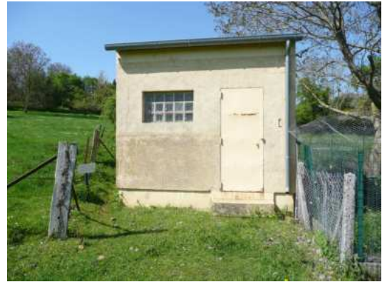
Station de pompage
